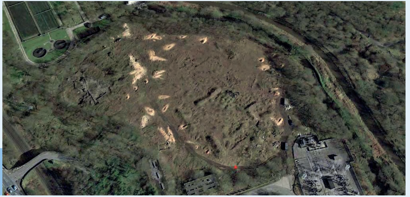
Aerial view of the power station site
